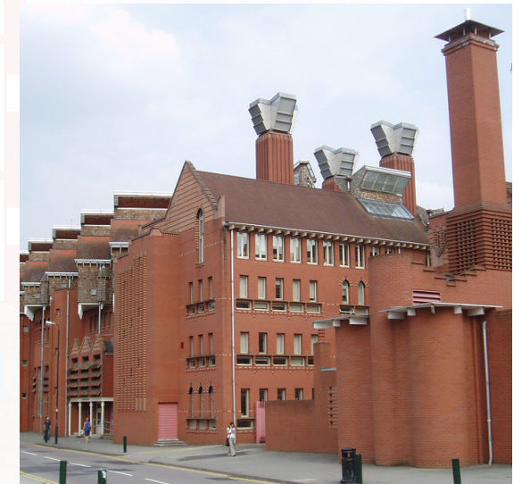
Windvanger Queens building de Montfort University - Leicester VK, architect: Short Ford Associates
